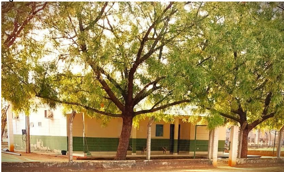
Figura 6 – UBSI-Gomes Carneiro – fachada
